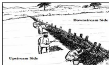
Fig.2. Single line simple weir.
